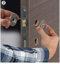
Put the handle roses together – and fitting is complete!
