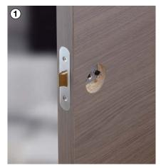
The enclosed black nylon sleeves are in place (though only in the case of lock holes of  $\emptyset$  8 mm)
