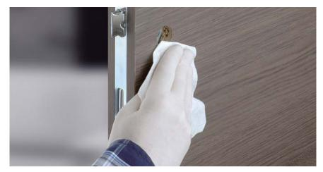
Clean the door surface in the area where the adhesive is to be used. Only the cloth delivered with the products should be used to clean or remove grease from the surface of the door. Smooth the protruding edges of the holes if necessary.
