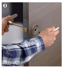
Put the door handles together and fitting is complete! (if necessary, stick on the escutcheons)
