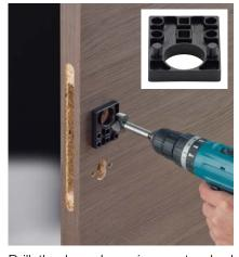
Drill the bore by using a standard Forstner bit (28 mm diameter) and the drilling jig available from HOPPE for the spring cassettes of flat handle roses.
